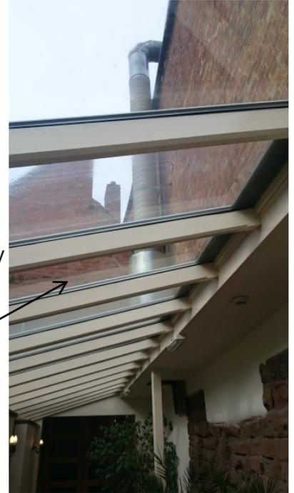
A conservatory has been built between two walls preventing access to the visible riser.
